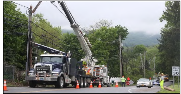
Figure 13. Central Hudson replacing a damaged utility pole following a severe storm (Source: Poughkeepsie Journal)
