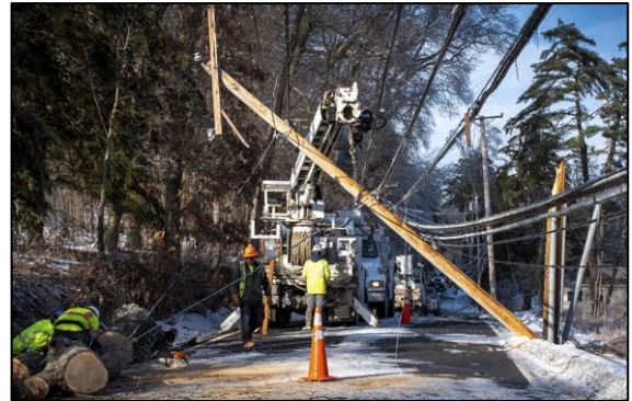
Figure 11. Central Hudson repairing a damaged utility pole blocking the road following a winter storm. Photo Source: Central Hudson.
